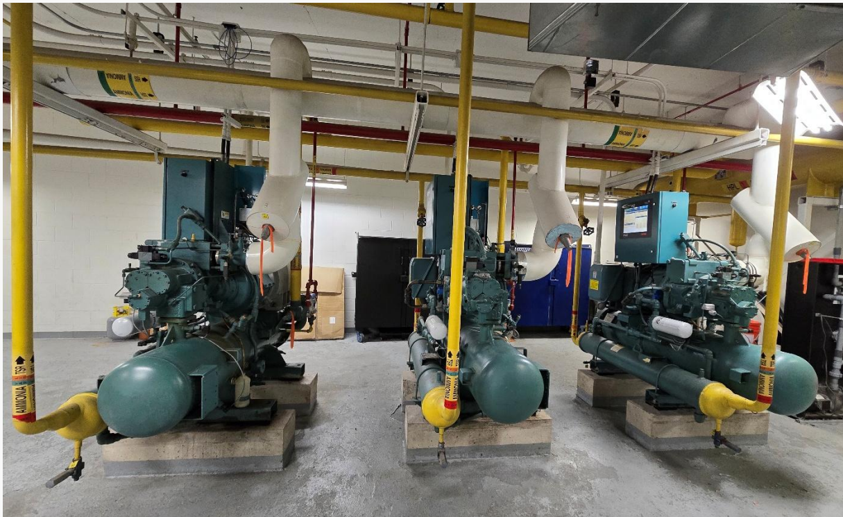
FIGURE 4.5: Three screw compressors in refrigeration unit
